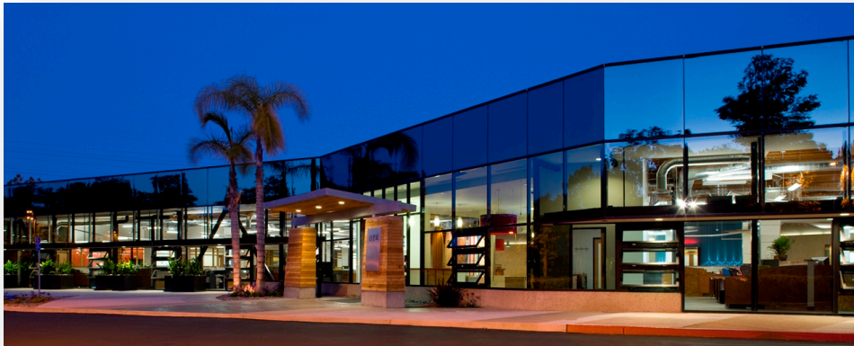
DPR Construction San Diego Corporate Office , Chip Fox, DG&E
